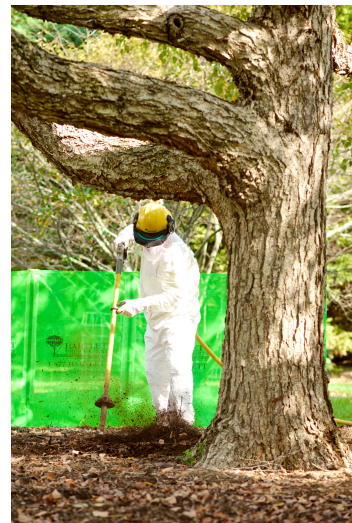
Figure 1: Soil decompaction using an air tool
