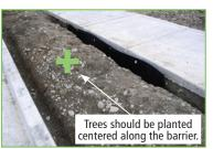
Roots may grow over the top of barriers set too low as well as through openings made for utilities or irrigation. An arborist review of the site details and tree species can help ensure effective and proper application of root barriers.
